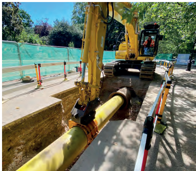
The pipe pusher in action on the Hyde Park project.
