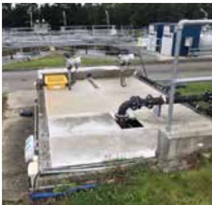
Off-Loading Point of Liquid PACL Sludge at the Purcellsinch Wastewater Treatment Works.
