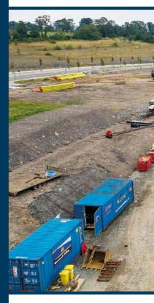
the existing network, providing a critical boost to the existing gas infrastructure in Dublin. This outlet pipework included a HDD underneath the M50 at one of its widest points across the main carriageway and both slip roads and was approx. 250m long through brown granite.
