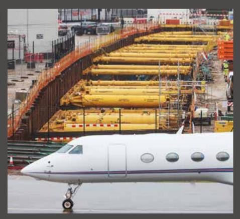
an open excavation has been avoided by installing a roof slab over the underground facility before commencing excavation.
