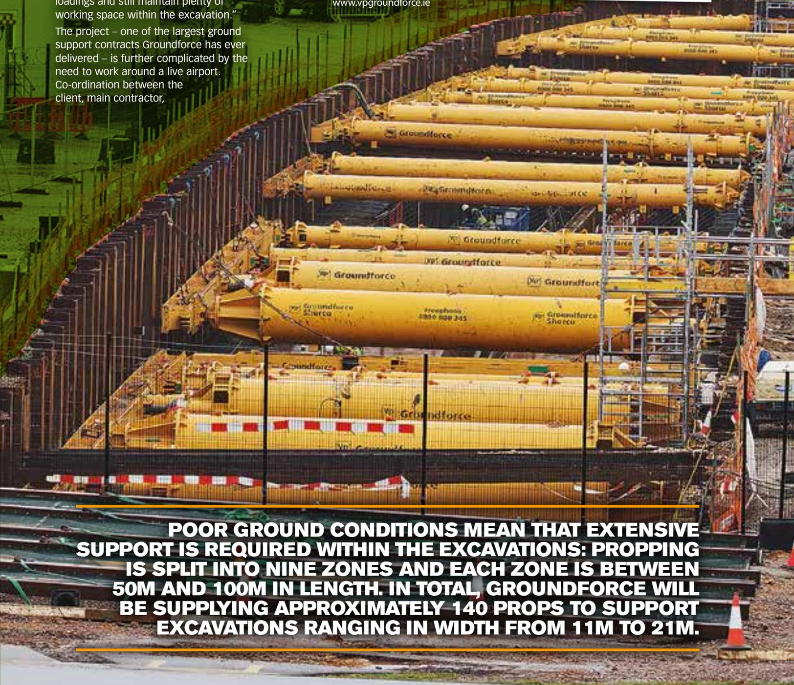
**POOR GROUND CONDITIONS MEAN THAT EXTENSIVE SUPPORT IS REQUIRED WITHIN THE EXCAVATIONS: PROPPING IS SPLIT INTO NINE ZONES AND EACH ZONE IS BETWEEN 50M AND 100M IN LENGTH. IN TOTAL, GROUNDFORCE WILL BE SUPPLYING APPROXIMATELY 140 PROPS TO SUPPORT EXCAVATIONS RANGING IN WIDTH FROM 11M TO 21M.**
