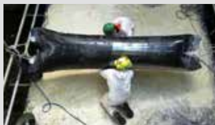
Pillow Packer Utilised to complete the works.
