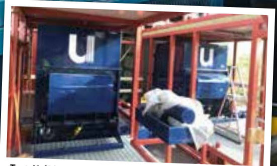
Two U-45LB Shredders being installed at L&T's Hämeenlinna oil filter recycling plant.
