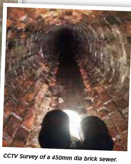
CCTV Survey of a 450mm dia brick sewer.
