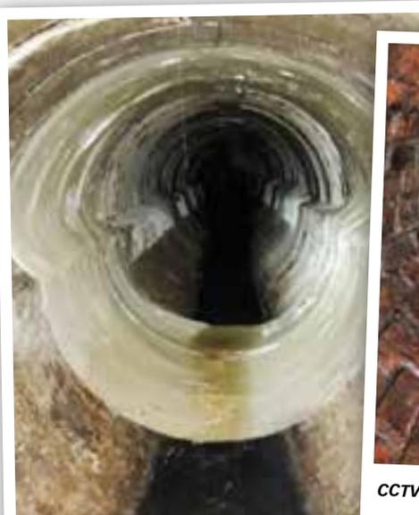
CIPP Patch Repair of 1440mm Dia Concrete Pipe.
