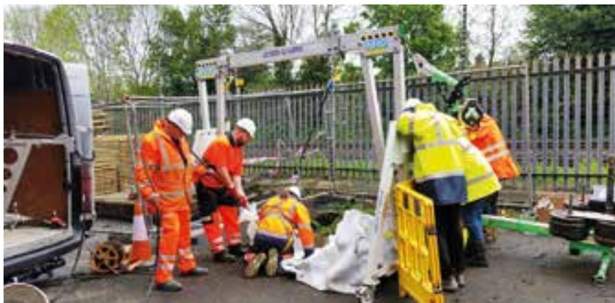
*The installation of a liner under railway tracks, we were able to repair the entire length of a pipe without affecting the railway lines at all.*
