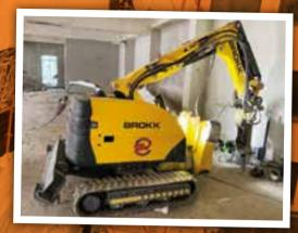
diggers and long reach machine with breaker, shears and muncher attachments. All materials from the soft strip – including timber, plasterboard, metal, glass and general demolition debris - has had to be carefully segregated and then transported from the site on artic and rigid trucks to recyclers and waste management companies across the country for reprocessing or disposal.
