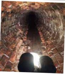
CCTV Survey of a 450mm dia brick sewer.
