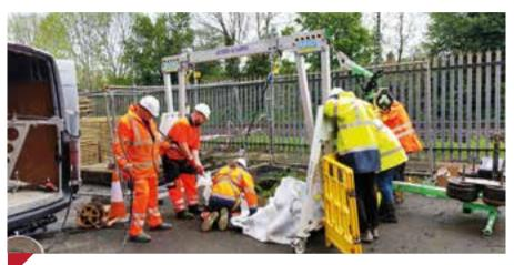
The installation of a liner under railway tracks, we were able to repair the entire length of a pipe without affecting the railway lines at all.
