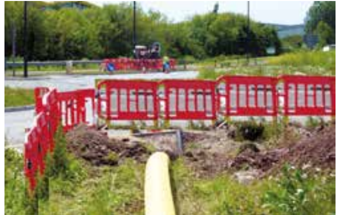
GMAC Utilities Ltd using a Ditch Witch JT30 Horizontal Directional Drill, installed 100 meters of a 250mm Gas Main under a roundabout in Avonmouth, Bristol.
