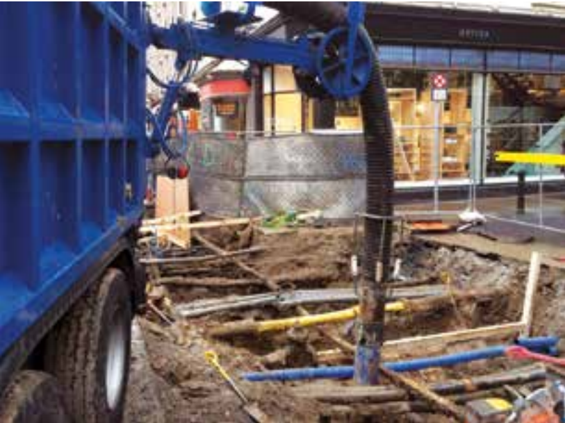
This photo was taken at a recent vacuum excavation between multiple utility services in Dawson Street, Dublin. These works are continually being carried out to facilitate works on the LUAS light project.
