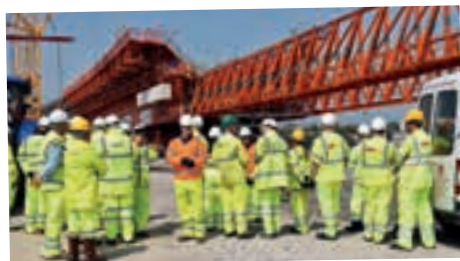
Looking at the £5m travelling former used for casting the deck spine.
